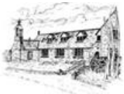
Marple Bridge (Hollins Lane)
